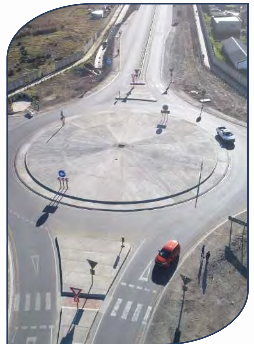
Rehabilitation of the Standerton Road
